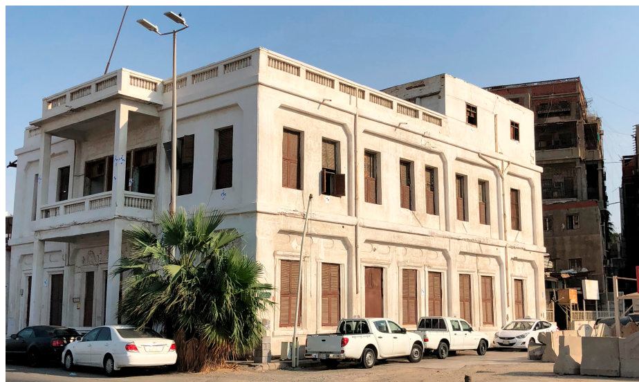
Figure 6. Bayt Zainal from the left-side elevation (west).
