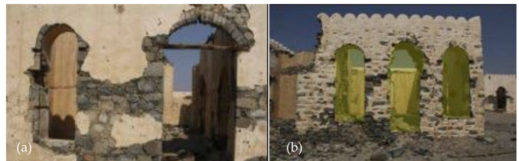
Figure 10. The palace in Ghiqa village: (a) shows window and door size ratio to wall, (b) shows window to wall ratio.
