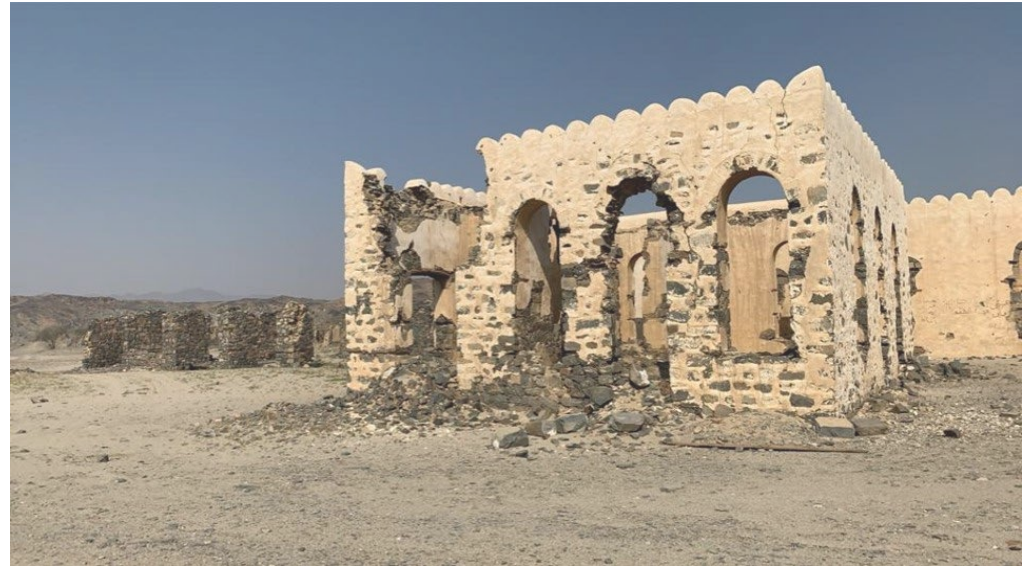
Figure 1. Historic Ghiqa Market buildings. The Ghiqa Historical Market, located in the Medina region of Saudi Arabia.
