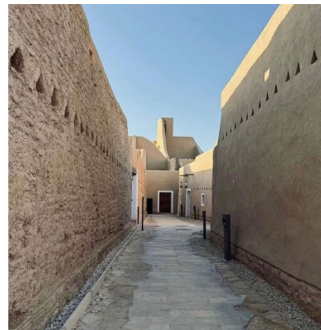
Fig. 7 Strategic placement of Alfuraj in Diriyah's transitional spaces, balancing light penetration and privacy
