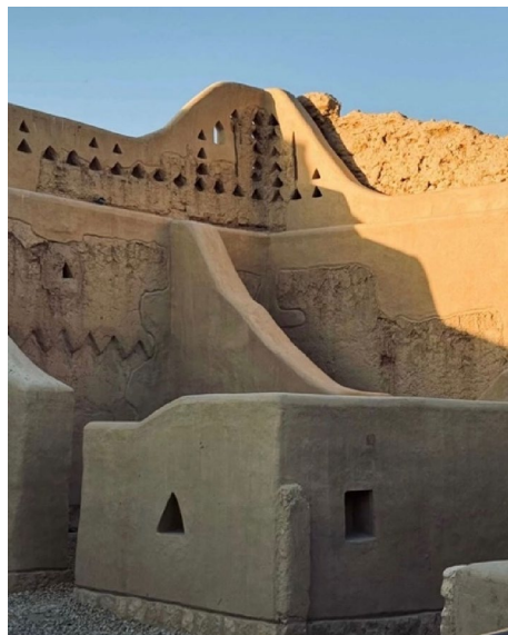
Fig. 6 Alfuraj configurations in Diriyah's traditional structures, emphasizing their role in environmental modulation and spatial identity
