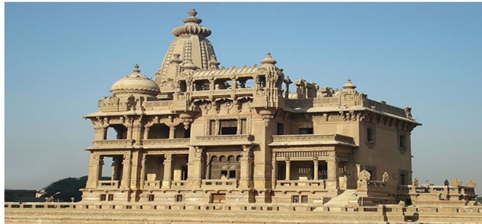
Figure 1. Baron Empain Palace in Egypt [19].
